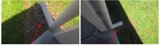
GuttersCorrosion in guttersGutter has corroded and require replacing. (Roof plumber)
