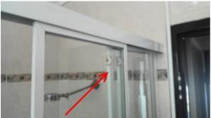
Shower tilesMouldy sealantMinor DefectType: AMouldy sealant between the junctions of wall and floor tiles in the shower area requires removal and<br/>replacing. (Tiler)
