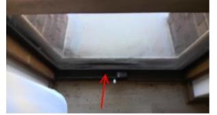
WindowsSash operationMinor DefectType: EWindow winder is missing and requires replacing. (Window manufacturer)
