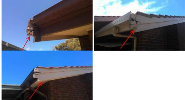
Downpipes Corrosion in downpipes Minor Defect
