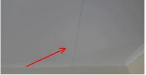
Ceilings Nails popping Minor Defect Type: A Sagging has occurred to the ceiling, which has caused the nails to pop from the ceiling lining, and requires re-fixing and repainting. (Plasterboard fixer and Painter)
