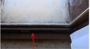
Doors and door framesDoor not closingMinor DefectType: EDoor is not closing correctly and requires adjusting. (Carpenter)
