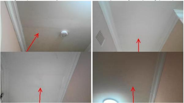
Cracking has occurred in the masonry wall, which is can be common in this type of construction this type of cracking is typical movement that occurs in the walls and the foundations and it can be repaired although the cracking will continue to reoccur overtime. (Engineer and Plasterer)
