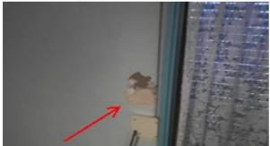
Back panel on the built-in robes is loose and require repairing. (Cabinetmaker)
