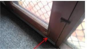
Doors and door frames Damaged door frame Minor Defect Type: A Door frame has been weathered and water damaged and requires repairing. (Carpenter)
