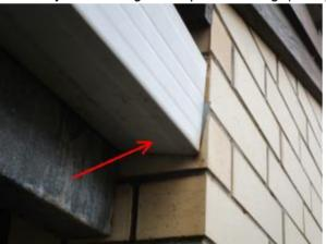
Mortar on the ridge capping is cracked and loose and requires re-pointing. (Roof tiler)
