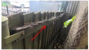
Property fencing Corroded fencing Further Investigation Type: A Boundary fence has corroded, and requires the corroded sheets replaced. (Fencing contractor)
